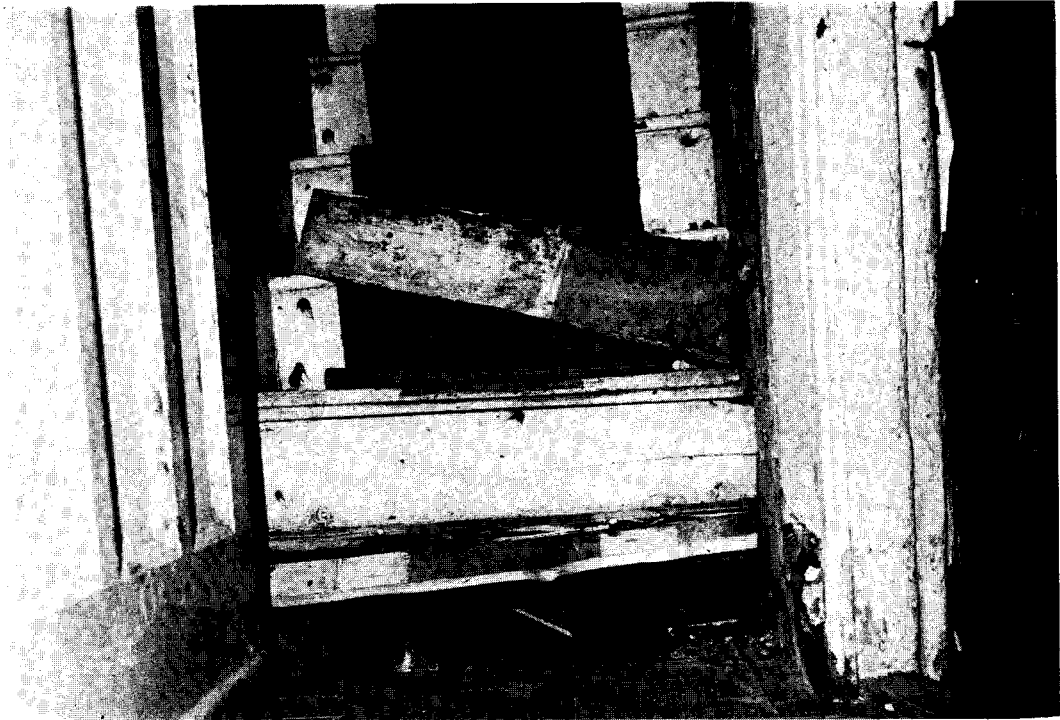
Wrecked staircase at 43 Mary Street
