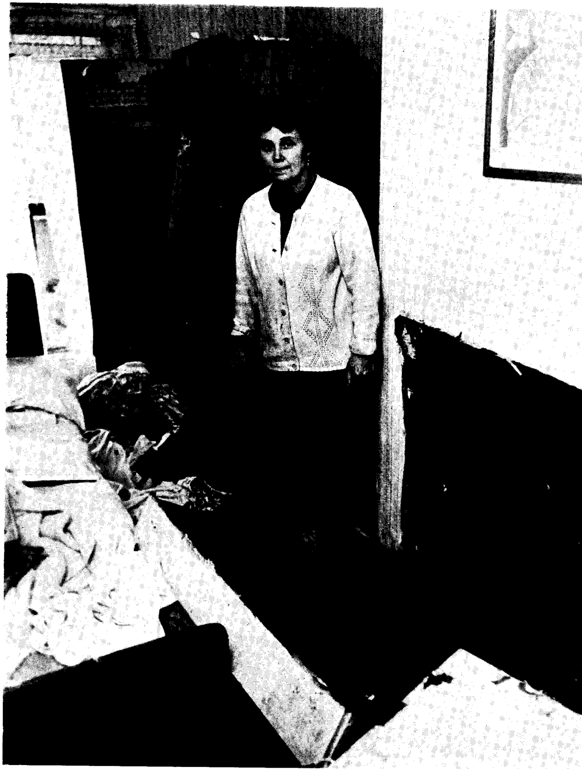
A wrecked bedroom with fireplace ripped out from wall at 90 Plevna Street
