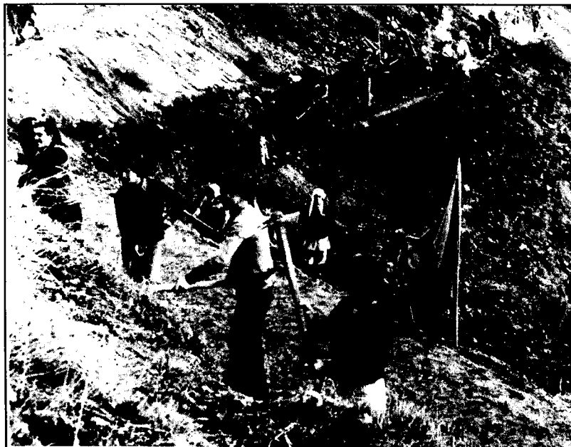
■ Youth Volunteers in a mass action to construct terraces
